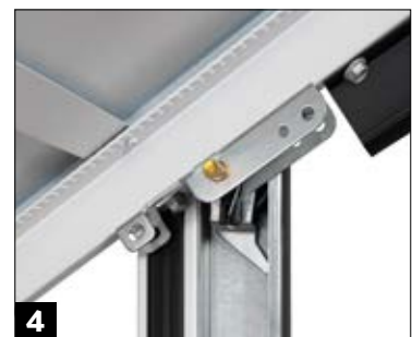
4 Guide rail & anti-drop safety mechanism
